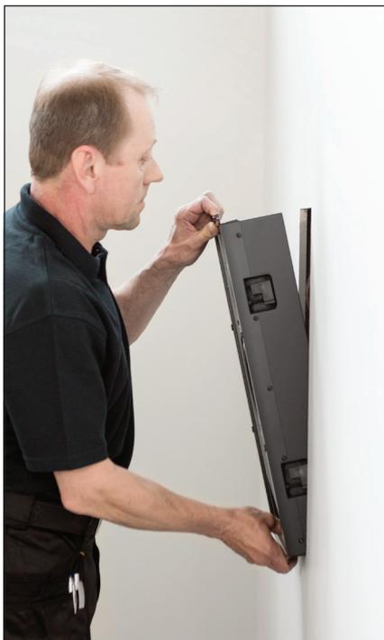
Figure 2. Lift the AIW26B enclosure into the hole.
