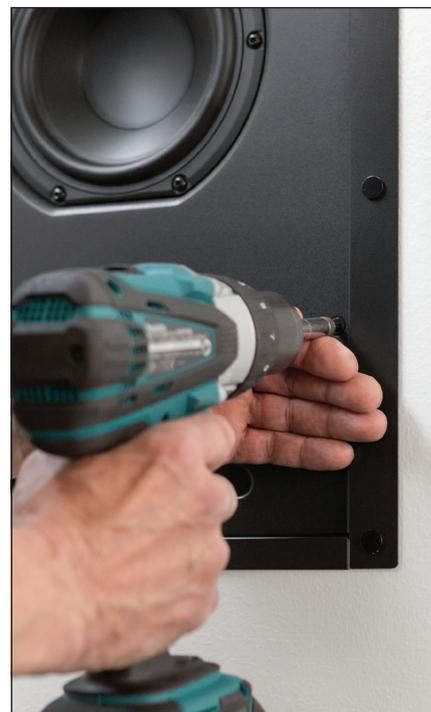
Figure 5. Tighten the four Torx T25 screws to 1.5 Nm (1.1 lb ft).
